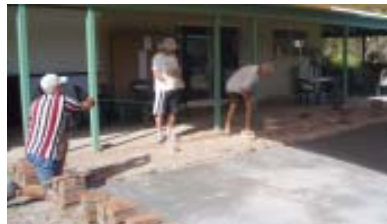
Praying the paving will look good
